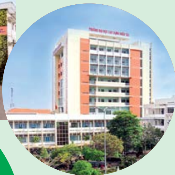
Mien Tay Construction University (source: mtu.edu.vn)
